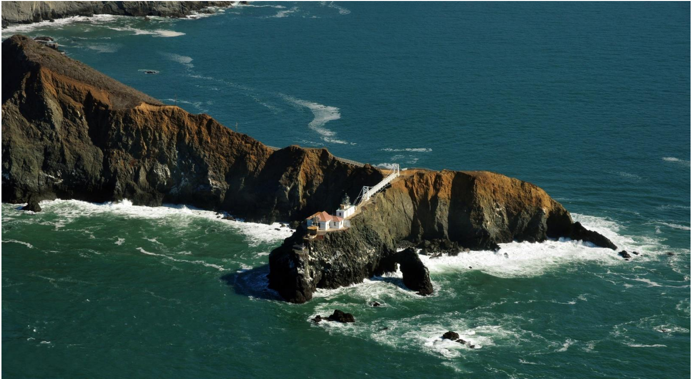
San Francisco Aerial photograph of the Point Bonita light house and light keeper's compound located on Marin headlands at the north end of the Golden Gate Bridge, taken from a Cessna 172 by Roger Bazeley AUXPA1.
