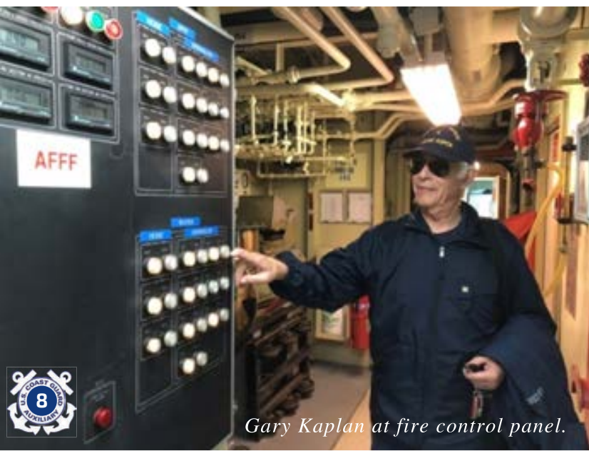
Gary Kaplan showing fire suppression foam making station.
