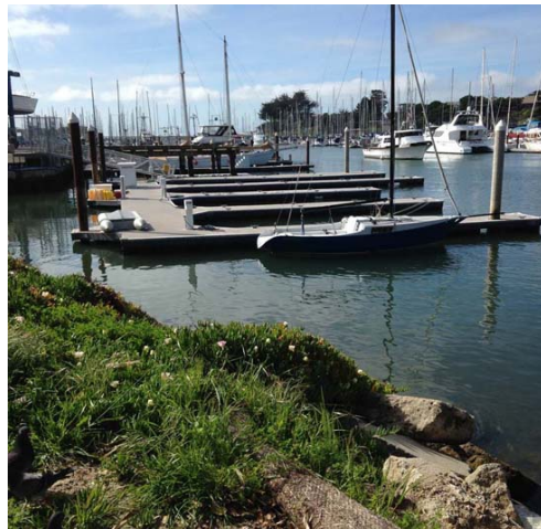
The Boatyard – all docks replaced!
