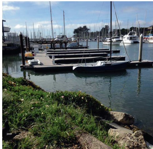
The Boatyard – all docks replaced!
