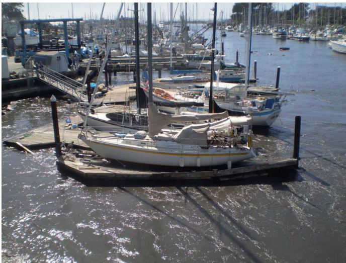
Tsunami flow tears docks apart at the Boatyard.
